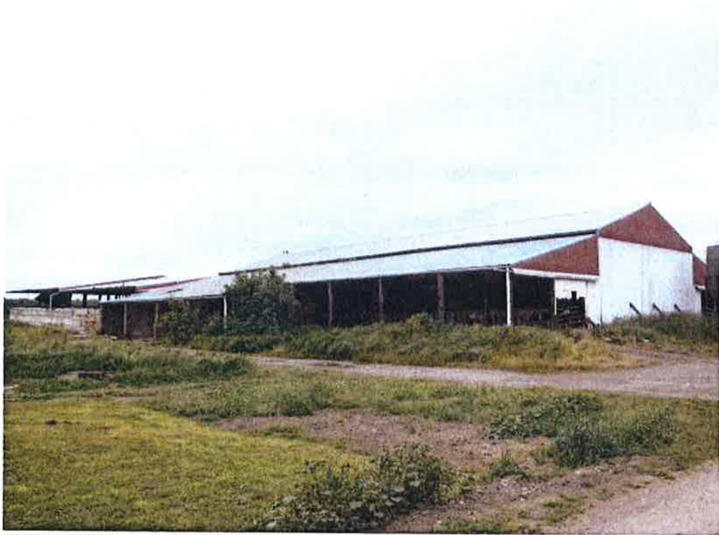
Old milking parlor (photo courtesy of Clallam County)
