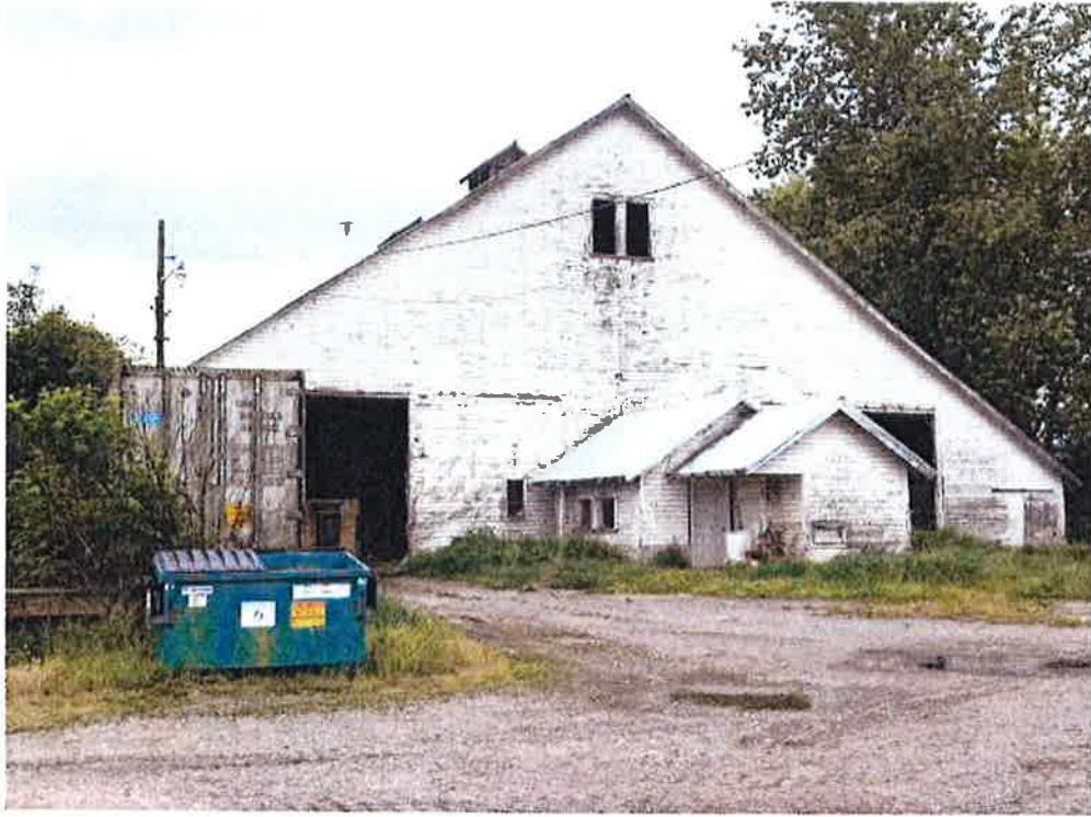
Large barn (photo courtesy of Clallam County)
