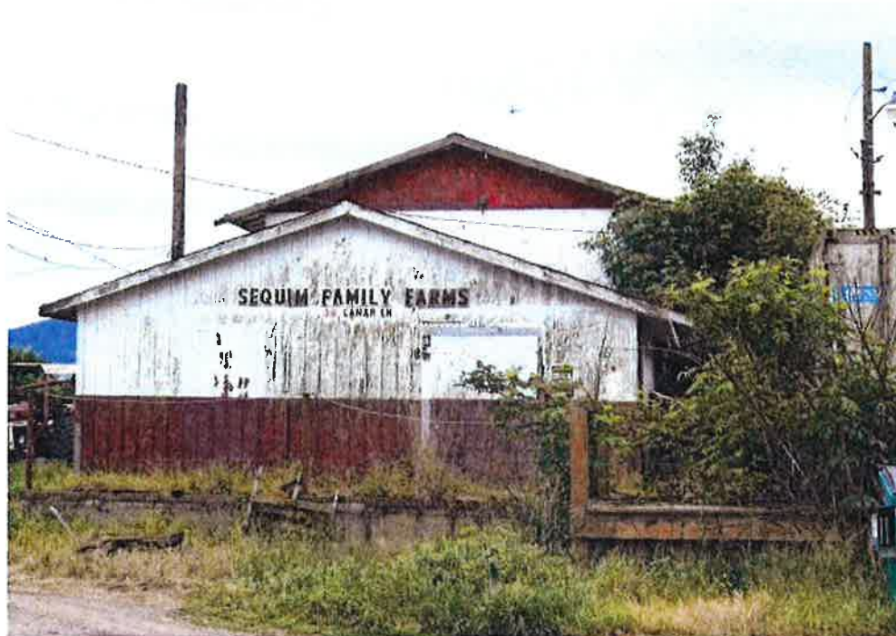
Refrigeration and creamery building (photo courtesy of Clallam County)
