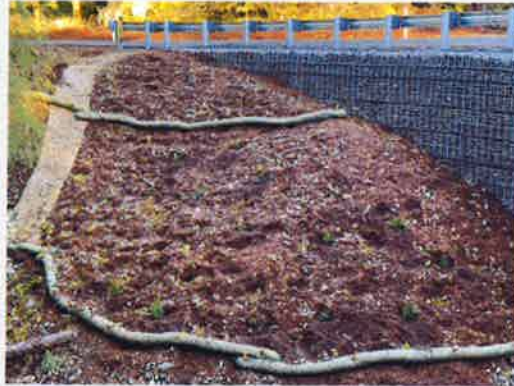
Planting the new culvert at Kugel Creek on Cooper Ranch Rd
