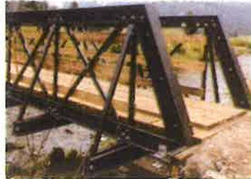
FRP Bridge with Sloped End Sections & Customer Supplied Timber Horizontal Rails
