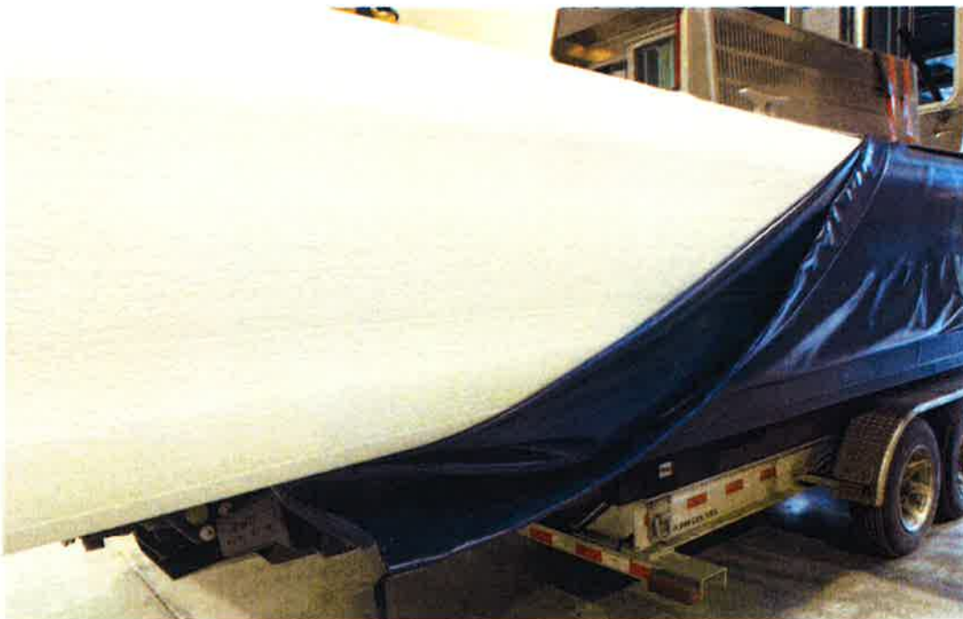
FIGURE 7: FOAM INSTALLATION INTO MEMBRANE
