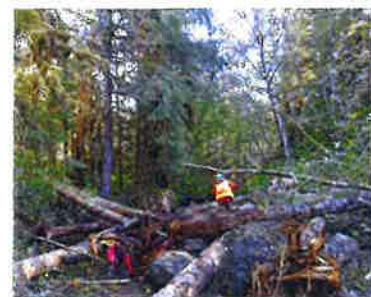
Above: The construction lead on the water climbs over logs and boulders as a Chinook helicopter installs more structure for the ELJ in Shale Creek. Wood and boulders are placed strategically to lock the wood securely, while still allowing enough water flow for fish to pass. Left: An established jam installed in 2021, about 200 yards downstream from the 2025 jams. In the past 4 years, this jam has formed a new large pool and gravel bar. Photos by Alex Bradberry
