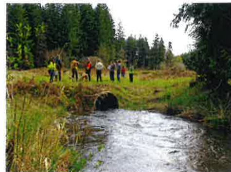
Fish passage barrier culvert at Ripple Creek before construction. Photo: Christa Bale
