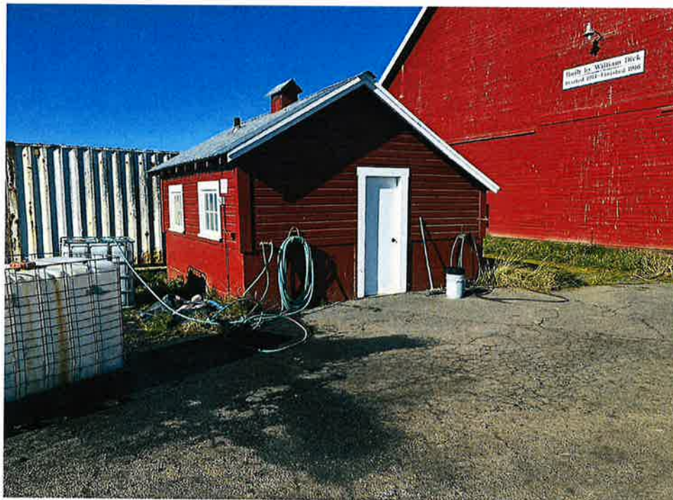
Former milking shed just south of the Barn. This is used as restroom facilities for the barn.
