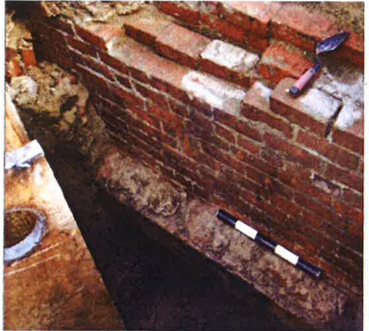
historic structure in SR99 tunnel
