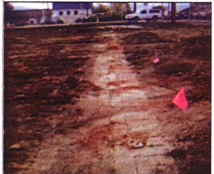
intact foundation below parking lot
