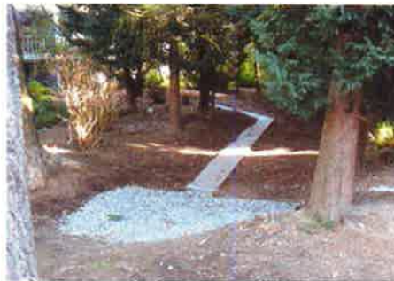
Infiltration trench
