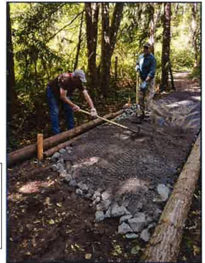
Spreading gravel layer.
