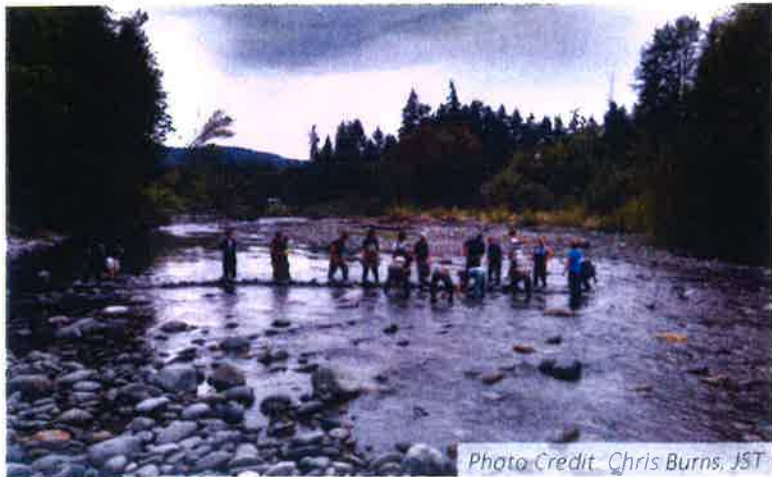
Crews installing rock dams in the Dungeness River to help fish move upstream during the 2015 Drought.
