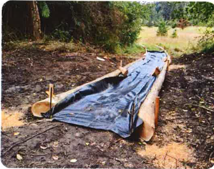
Construction of turnpike across a wet area.
