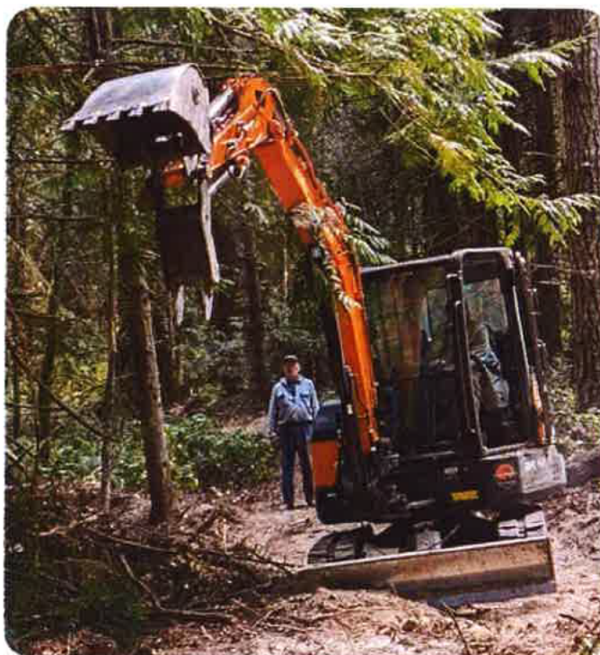
Dan Dosey operating excavator and Jim Hollatz assisting to refine trail tread
