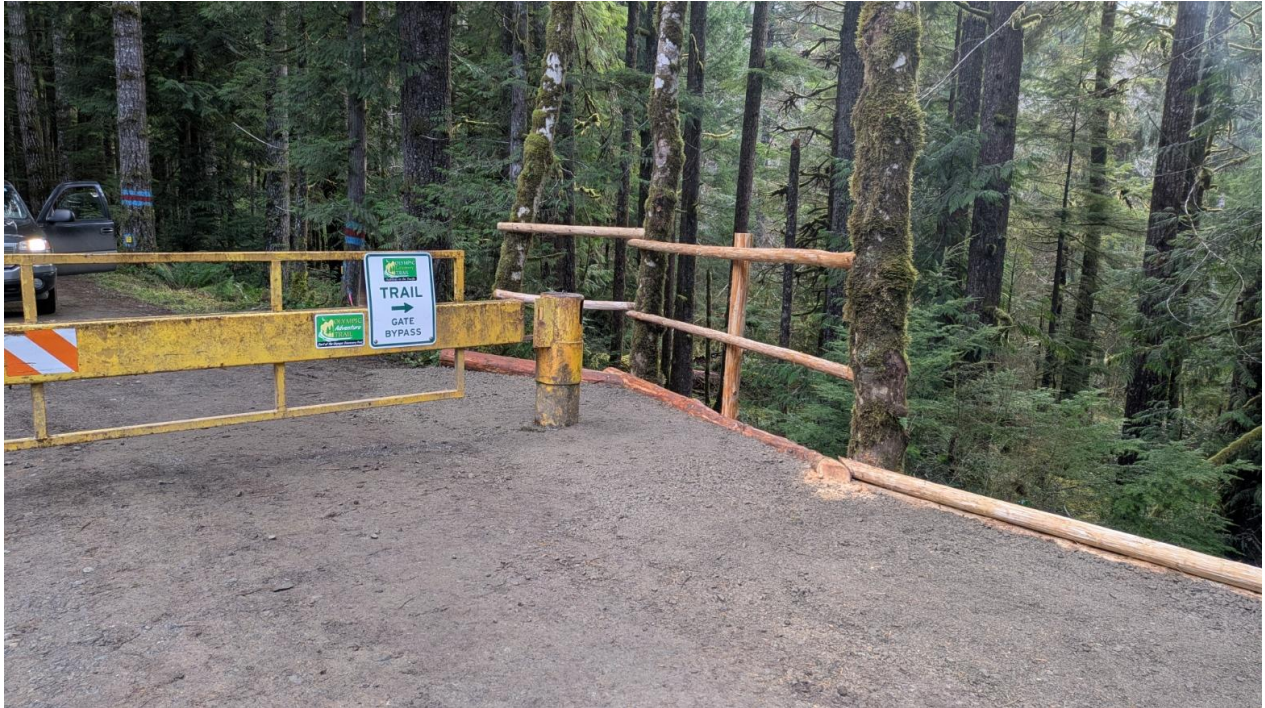
Waterline Road gate bypass Thank you Justin!
