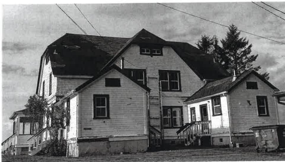
Keepers' Cottage looking north shingles missing after the first storms of Oct. 2024
