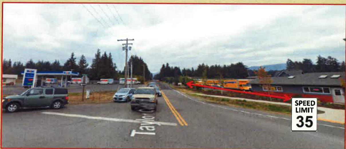
SAFELY Rated for 35 mph — Taylor Cut-off Road (Looking South from US 101)
