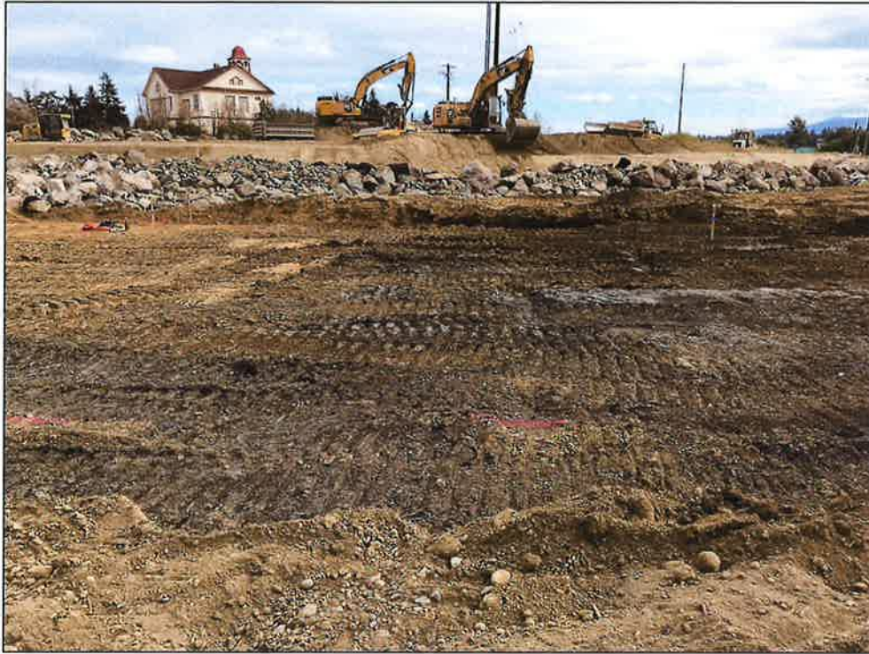
Looking east: flood return channel, key trench, levee, Dungeness Schoolhouse. 9.23.2022
