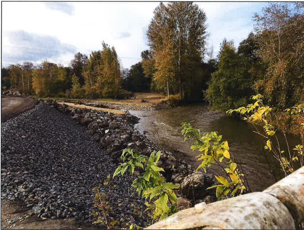
From Schoolhouse Bridge: Levee, flood return channel, Dungeness River. 10.31.2022
