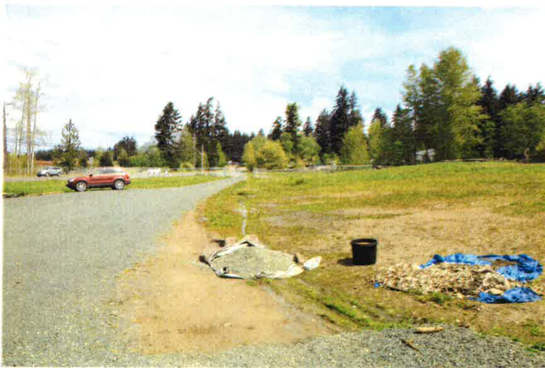
FIGURE 2: View of access road that enters the site from its north-east corner.
