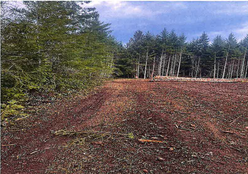
Image 1: Site of harvest/conversion activities. All stumps and vegetation removed from site. Site has been graded/leveled. Approximately 0.60 acres in size.
