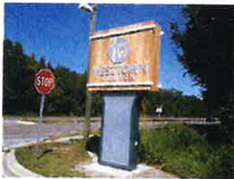
Pylon signs are erected on freestanding poles, which may be encased within metal cladding, such as this church sign. Photo provided by Creative Sign Designs.
