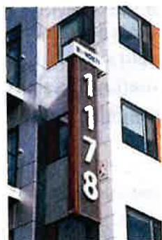
A blade sign is installed perpendicular to a structure. Some sign codes favor installing blade signs instead of those flush to the wall. Photo provided by ArtFX Signs.
