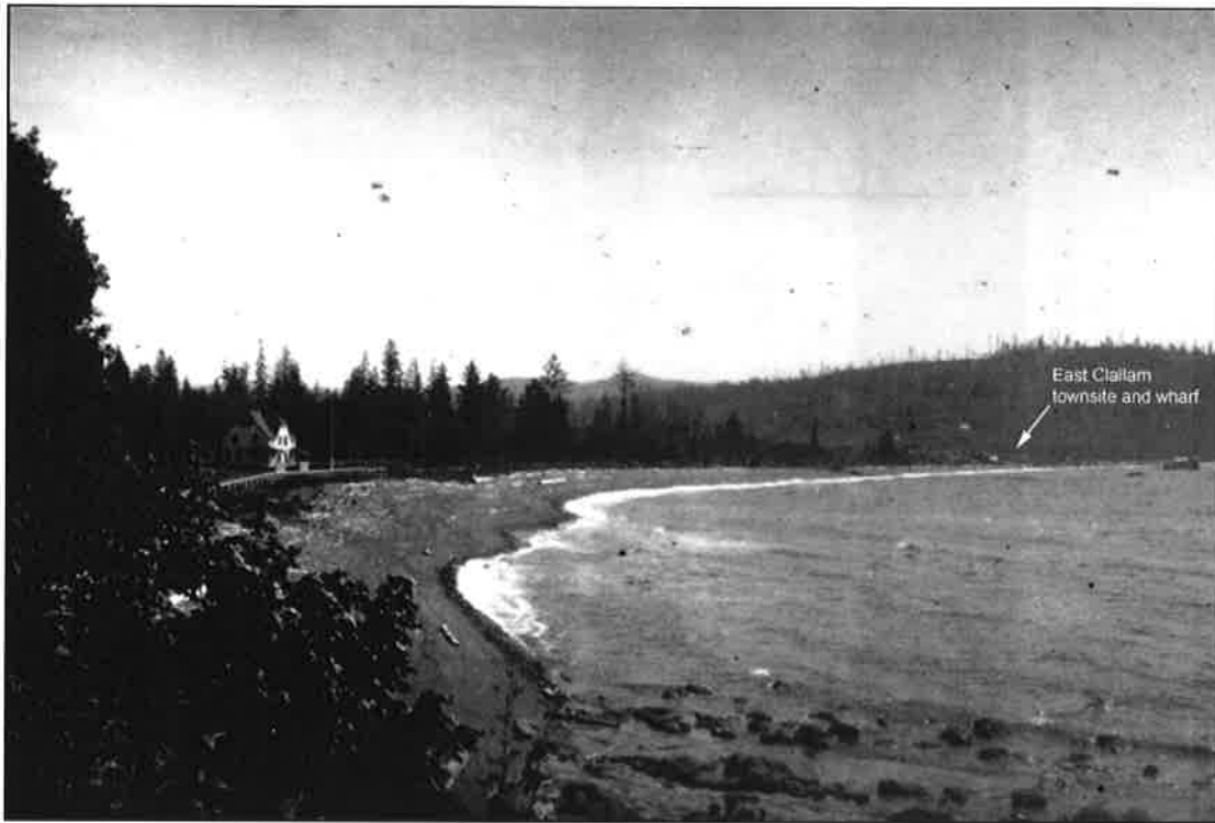
Figure 4. Slip Point Light Station Operations Area and coastline shortly after construction (Forks Timber Museum).
