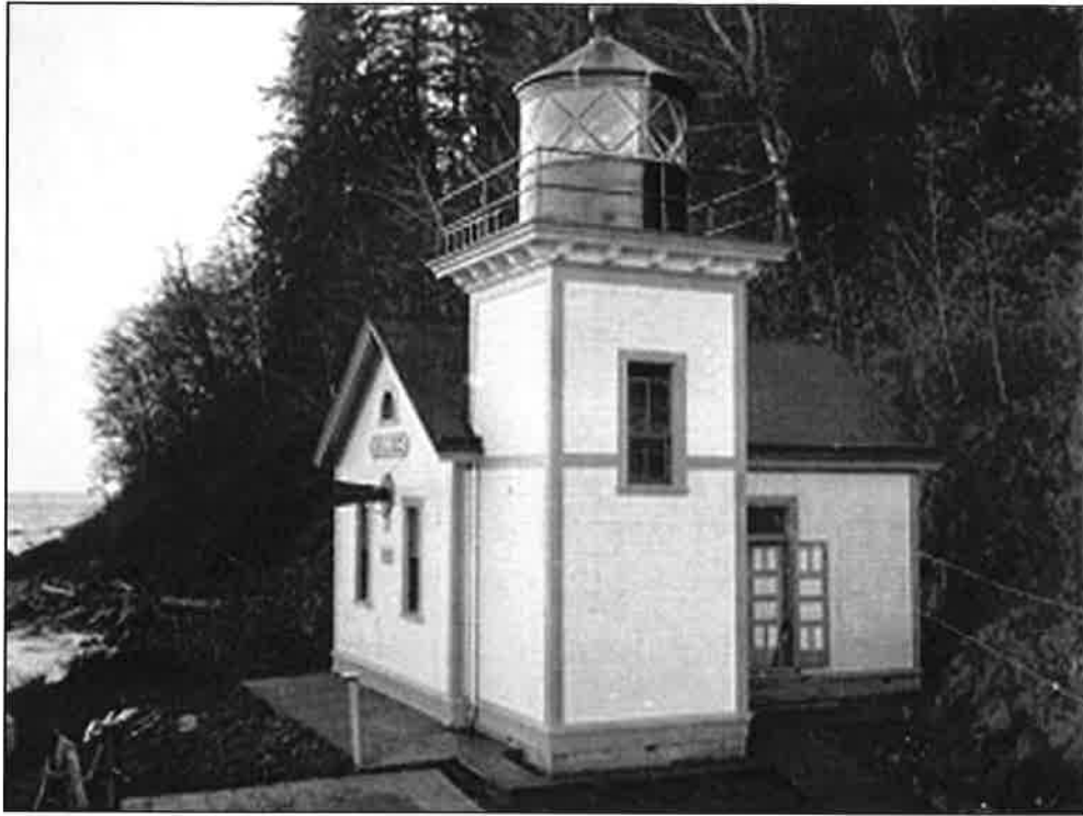
Figure 6. Remodeled Slip Point Light and Fog Signal Building about 1916 (USCG).
