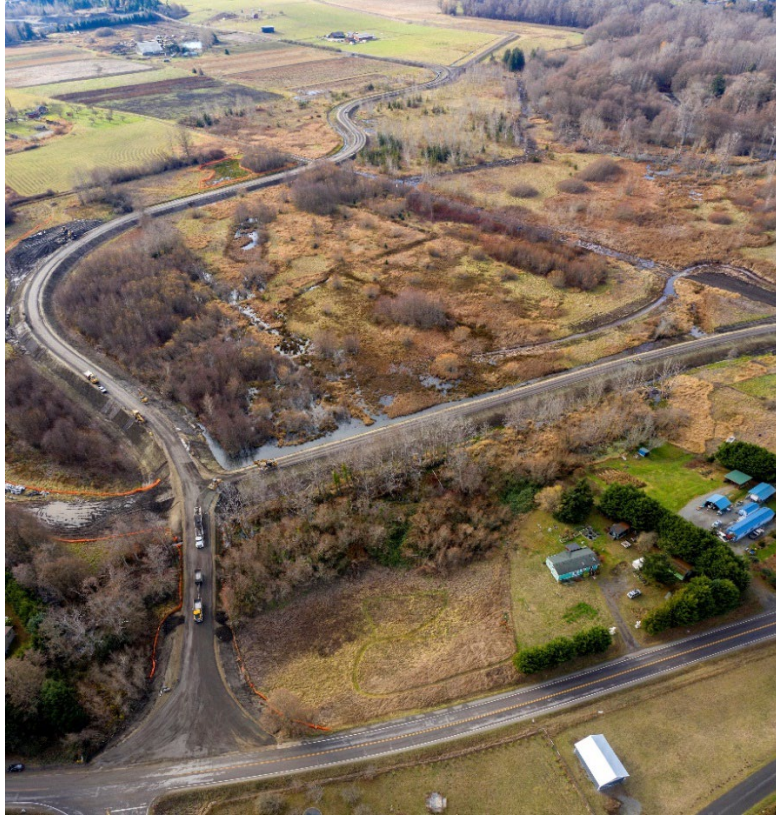
Overhead view of the newly constructed levee, taken north of the Lower Dungeness River Floodplain Restoration and Levee Realignment project site, looking south, in December 2022.
