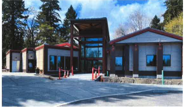
April 2022 as built; landscaping to come in May.
