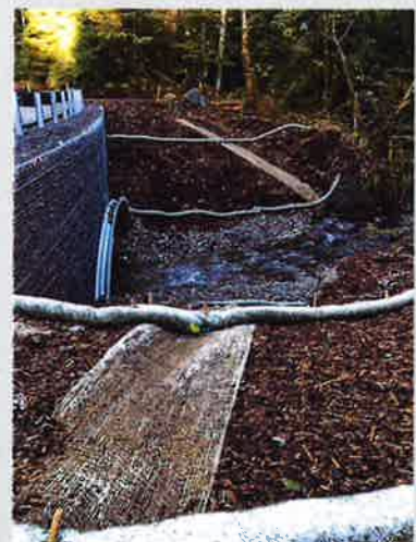
Kugel Creek Culvert replacement
