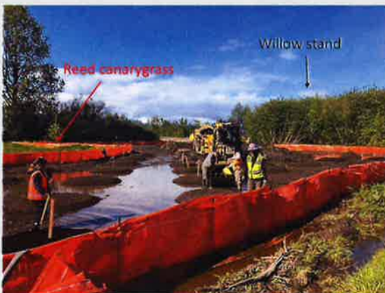
Reed canarygrass being scrapped and removed, hummocks being installed in May 2022
