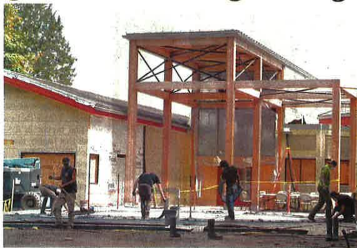
Construction continues at the newly-renamed Dungeness River Nature Center in late August. Workers with Hiday Concrete, Inc., work on the "patio" that will more than double the original outdoor entrance space, river center officials noted last week. The center, undergoing a multi-million-dollar expansion, is expected to reopen this fall. Sequim Gazette photo by Michael Dashiell
