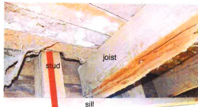
full 2" x 10" joists approx. 24" OC
