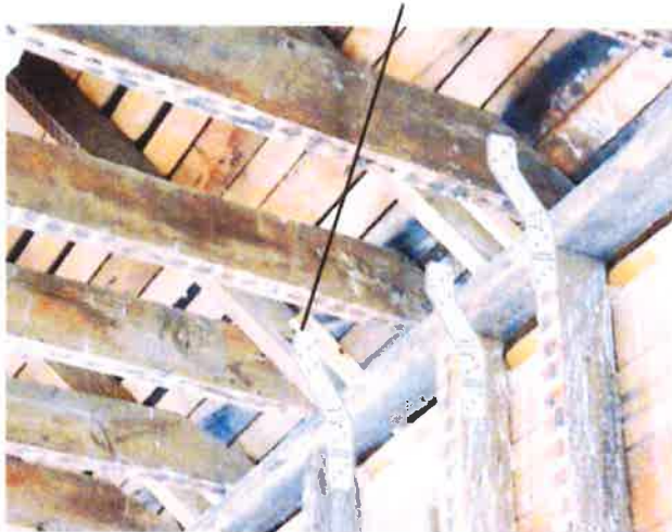
diagonal wire rope bracing make-up
