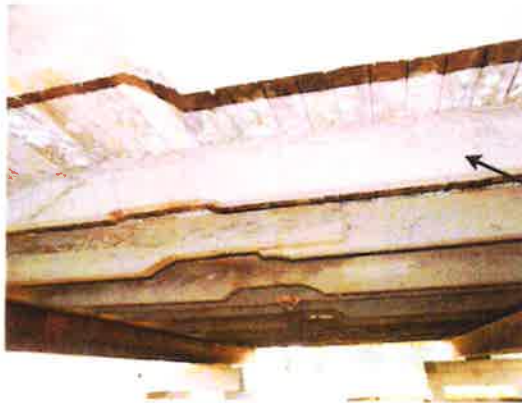
full 2" x 10" joists approx. 24" OC
