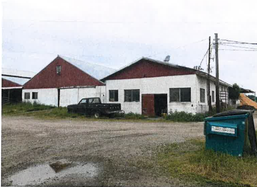
Cube barn, calf barn and free stalls (photo courtesy of Clallam County)
