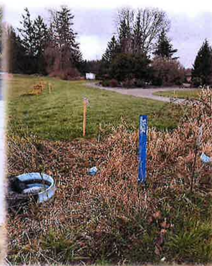
Dungeness Irrigation District piping
