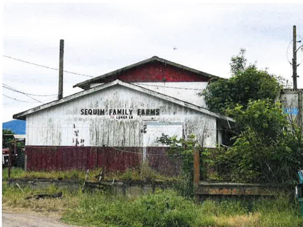
Refrigeration and creamery building (photo courtesy of Clallam County)
