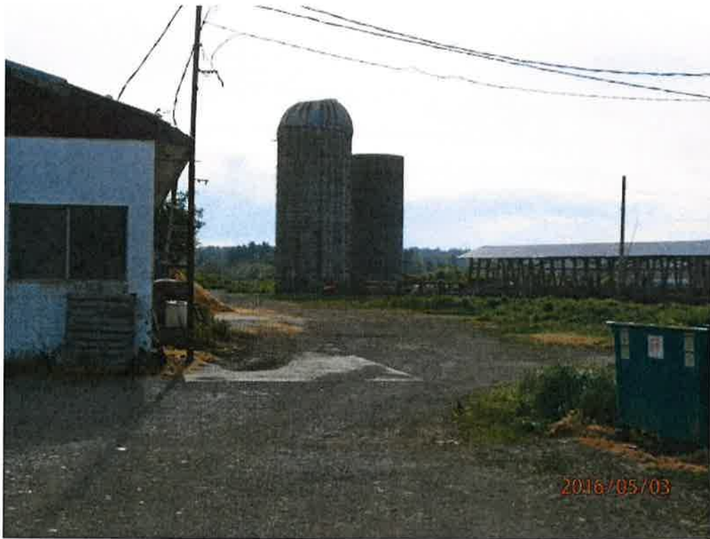
Silos (photo courtesy of Clallam County)
