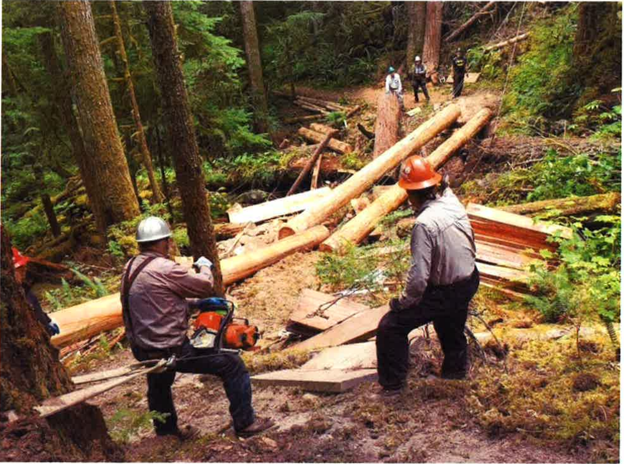
Slab Camp stock bridge
