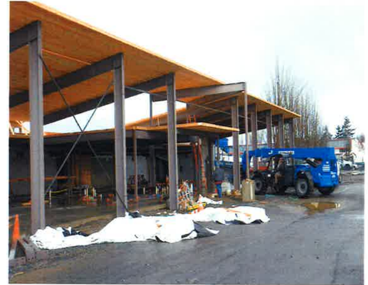
CLT for roof at Shore Aquatic Center
