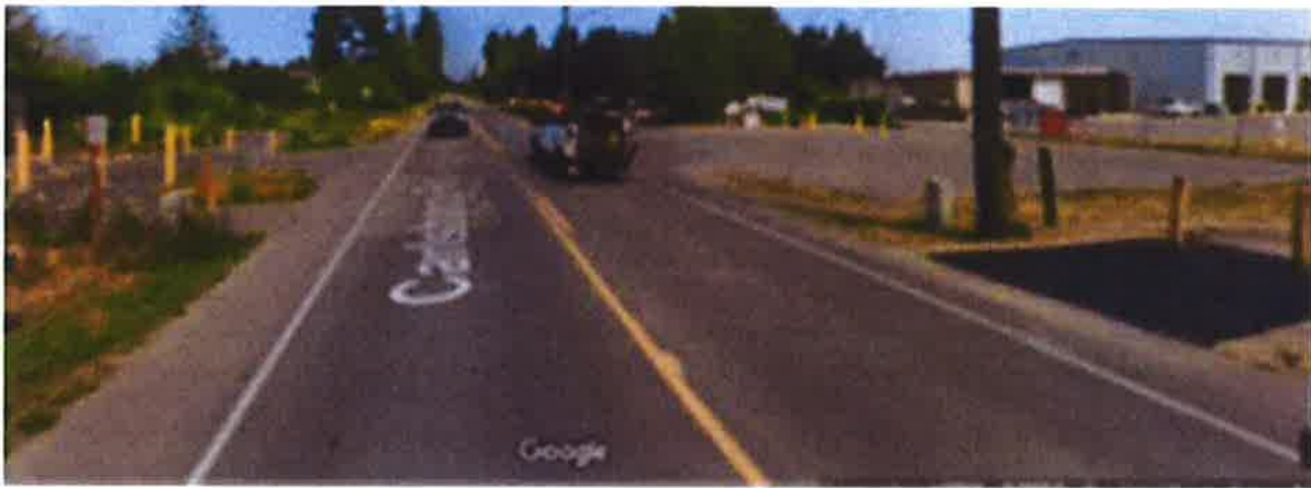
Existing Conditions looking north, ODT trail heads (East-West) visible.
