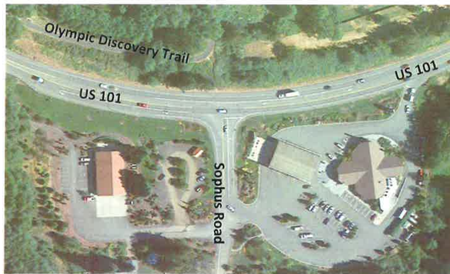
Figure 1-2. Existing US 101/Sophus Road Intersection
