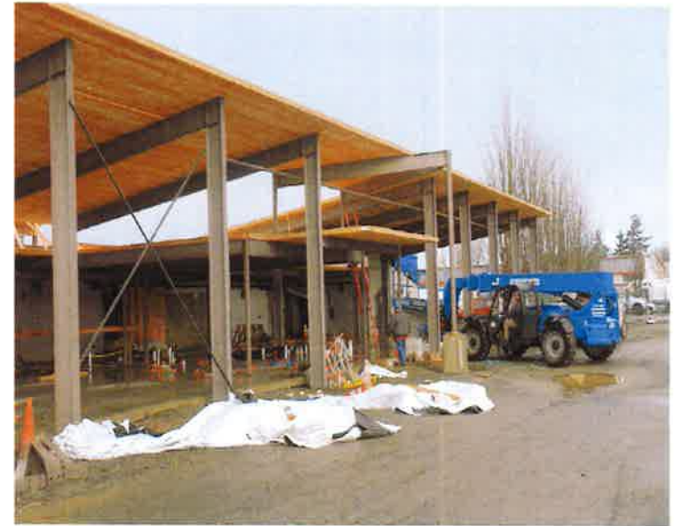
CLT for roof at Shore Aquatic Center
