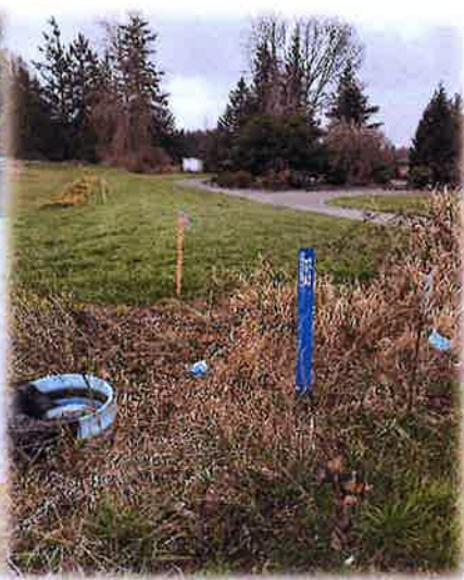
Dungeness Irrigation District piping
